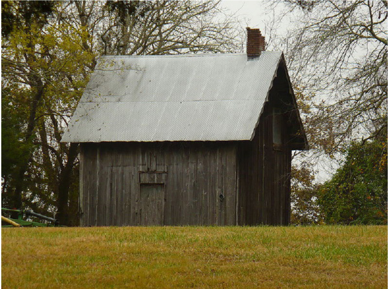
Figure 6. Faunsdale Plantation slave quarter, Marengo County, Alabama. Altairisfar, “Detail of one of the slave quarters, built in the Carpenter Gothic style,” December 31, 2007, photograph, accessed December 1, 2018, https://commons.wikimedia.org/w/index.php?curid=5309557 .
