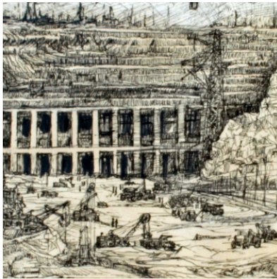
Electricity Station at High Dam
