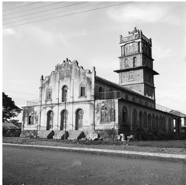
Fig. 2 Qde-Omu Central Mosque. Note the absence of domes and balustrades which were a later addition. Photo by Pierre Verger, ca. 1950s, © Fundação Pierre Verger.
