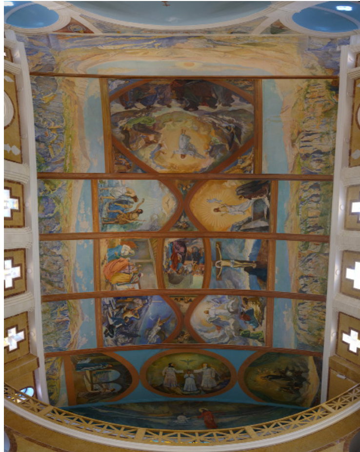
Full view of ceiling.
