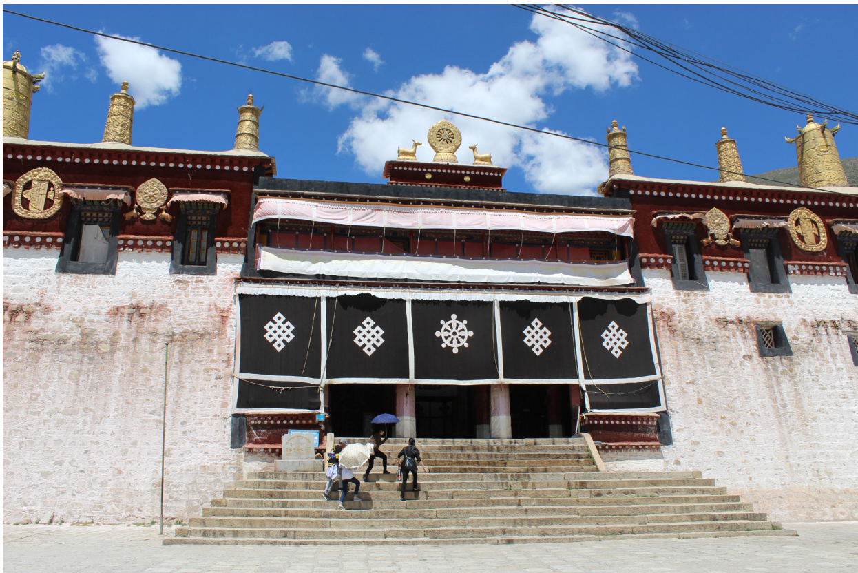
Fig. 4 An assembly hall at Drepung Monastery outside Lhasa, Tibet, with whitewashed stone construction, a penbé (Tib. span bad) frieze along top, distinct inset windows framed in black, and a flat roof, 2019. Photo by author.
