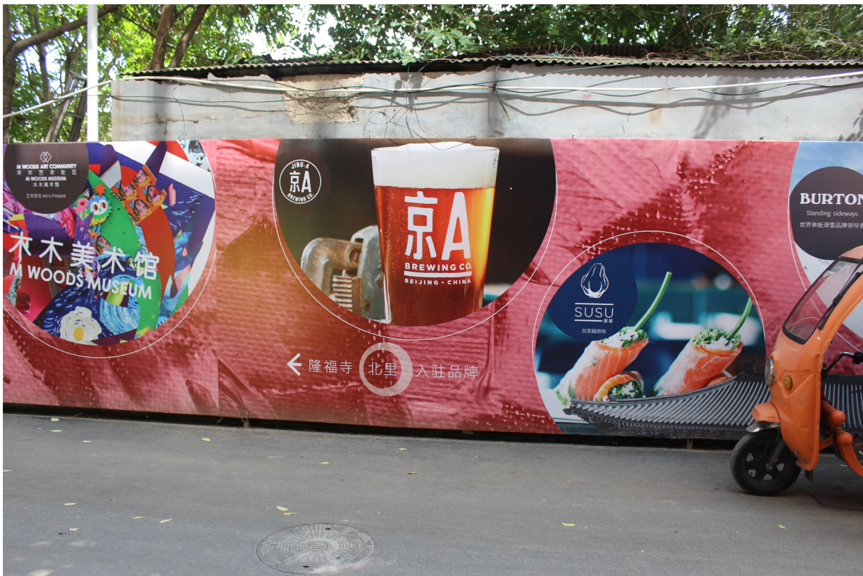
Fig. 28 Large ads covering the fencing around a construction area of the Abundant Fortune Temple complex displaying the commercial tenants that would be anchoring the space, 2019. Photo by author.
