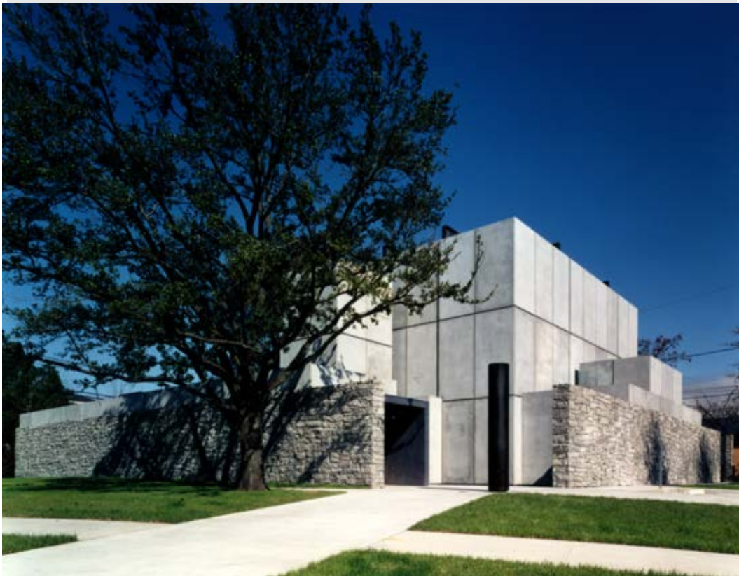
Exterior view of the Byzantine Fresco Chapel. Photo courtesy of and © Paul Warchol Photography.
